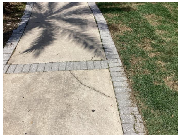
Sidewalk cracks
