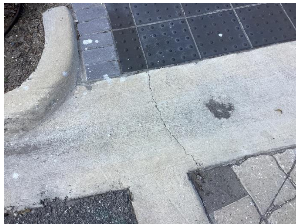
Concrete cracks
