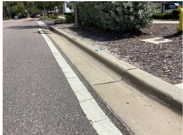
Concrete curb and gutter
