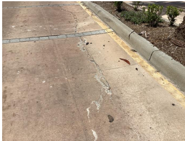
Street full depth cracks
