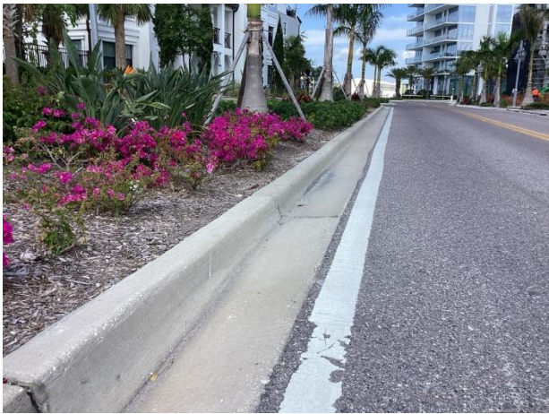
Concrete curb and gutter
