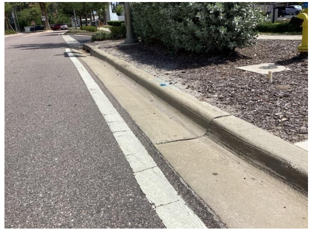
Concrete curb and gutter
