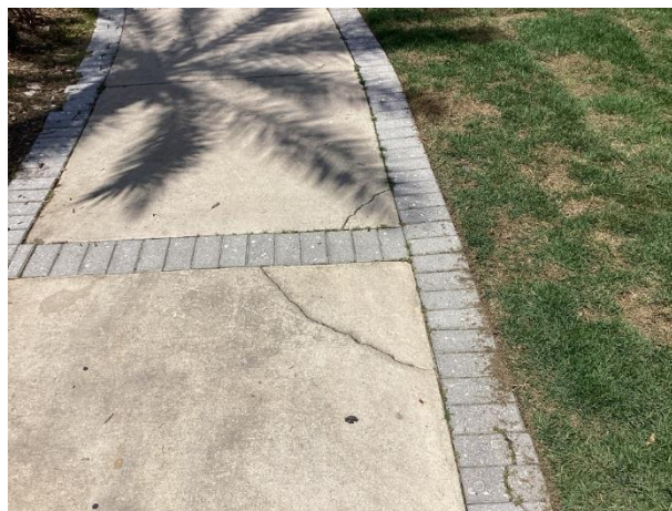
Sidewalk cracks
