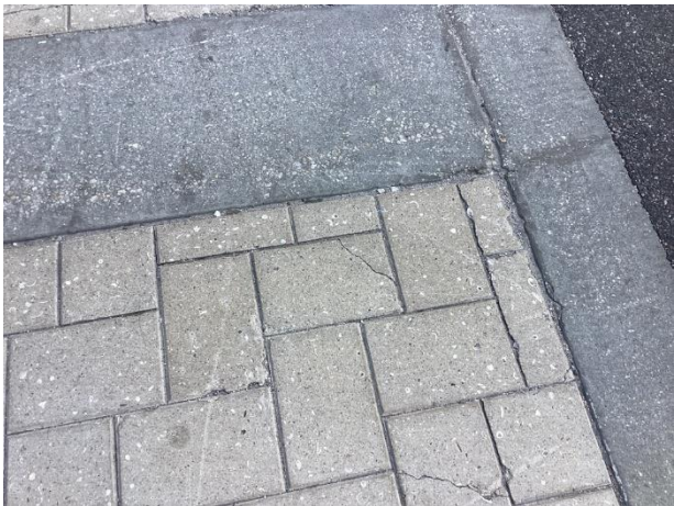
Paver cracks
