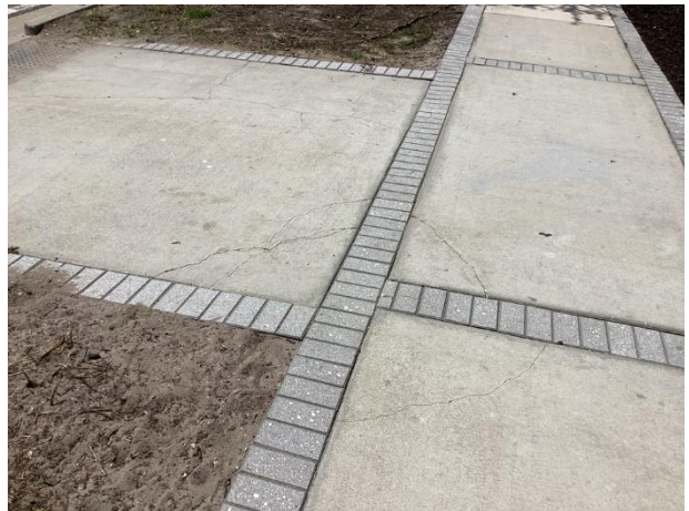
Sidewalk cracks
