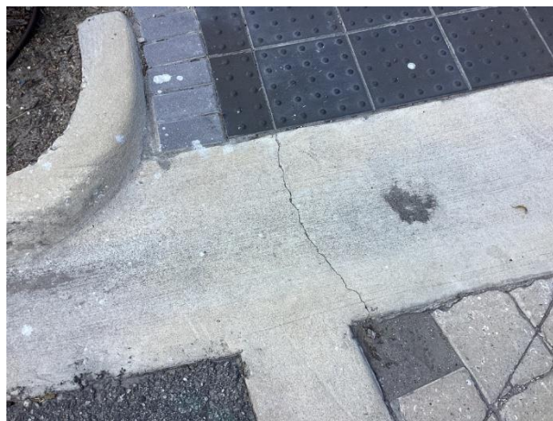
Concrete cracks
